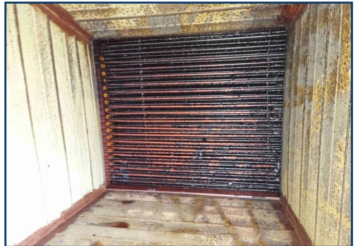
Internal view of the Lepido® from the exhaust inlet side after 22 months
